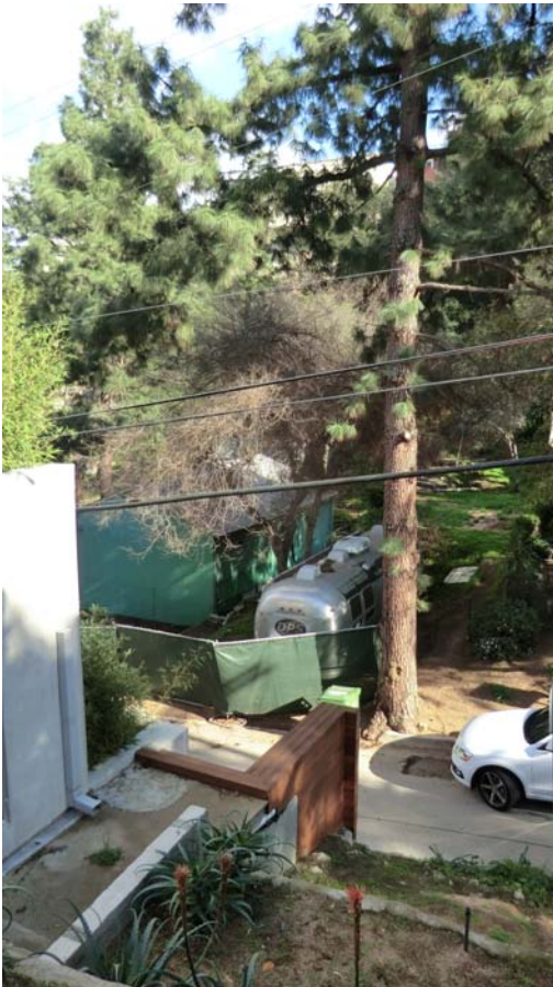
Note inadequate fencing of project site.
