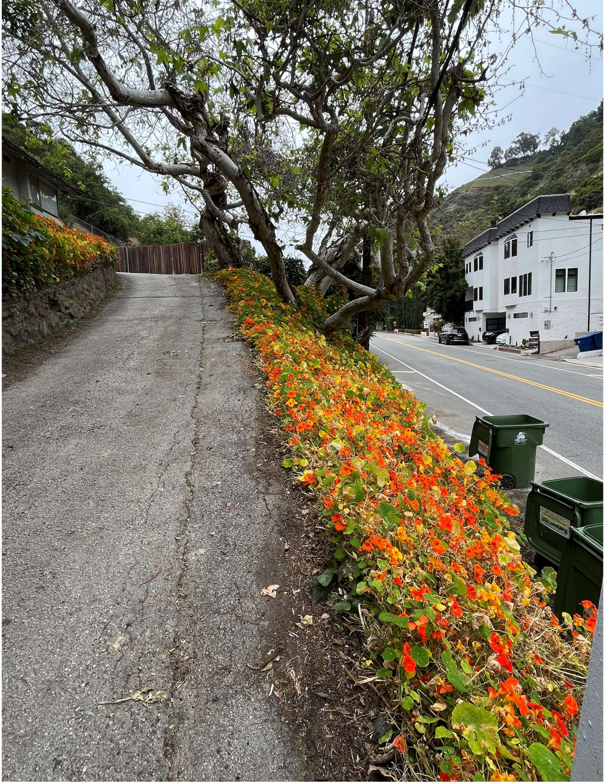
ANOTHER VIEW/PERSPECTIVE OF THE ENTRANCE TO THE PRIVATE DRIVE/EASEMENT HILLSIDE SUPPORT AND RETAINING WALL, NARROWING FROM THE ENTRY WAY TO APPROXIMATELY 11'. (THE EASEMENT IS 9' IN WIDTH.)
